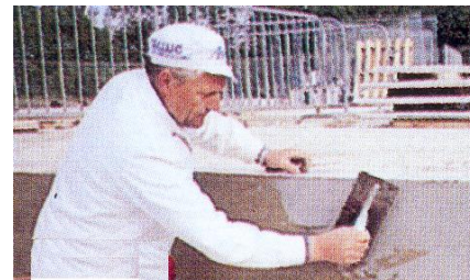
C106-05: Waterproofing Rendering
