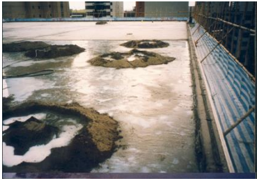
C106-05 : Waterproofing Screed on Roof
