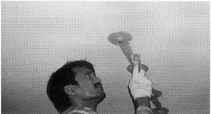
Seal the crack line with MP epoxy putty.
