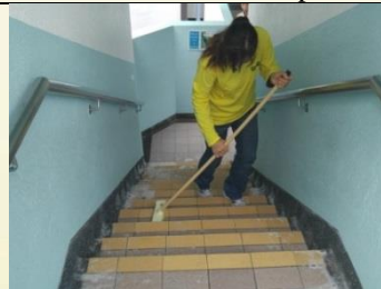
(2) Use appropriate tools to clean the floor by F223.
